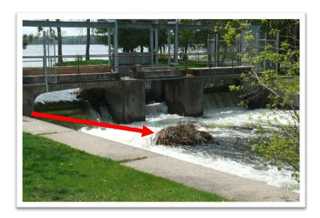
There was a second mass of vegetation (red arrow) located downstream of the eastern bay of the dam (below the dam) which was the remnant of a blockage that cleared earlier. This triggered the recent drop in water level that began after May 4<sup>th</sup>. A portion of this mass was still visible for some time after that date and was lodged on the top of the stop-logs of the eastern bay of the dam.
