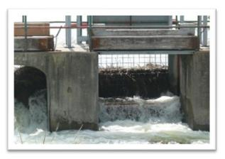
Recently a large mass of wetland vegetation was lodged in the central and eastern bays of the dam. The central bay with stop logs set to three feet acted as the main discharge point. However, a mass of vegetation was blocking this discharge keeping waters unusually high.
